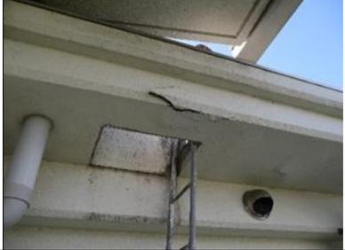
A photograph showing a close-up of the base of a building's exterior wall. A dark, irregular crack is visible in the concrete or masonry surface. To the left, a white vertical pipe is partially visible. The background shows a clear blue sky. | 東館北側の庇部分に割れが確認された。 |
